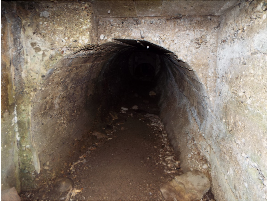
The flume (circa 1912) is accessible, leading to...
