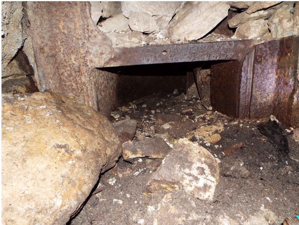
the entrance to the turbine.
