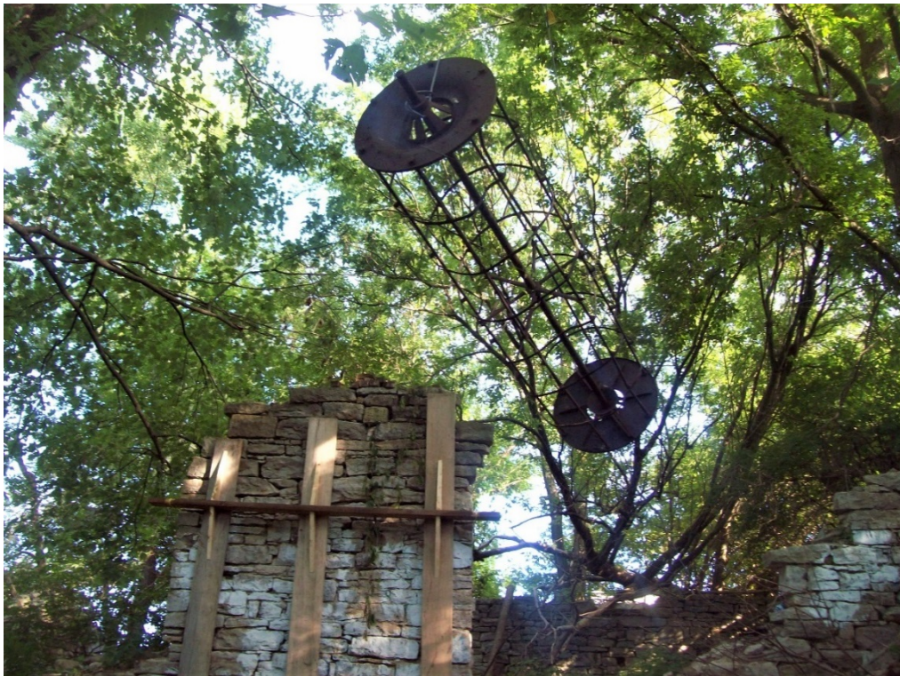
Top photo by Jack Harvey shows the boom truck from G C Hudson Supply that removed the machines where we needed to dig. Lower photo by Michael Whittaker shows one of the reels from a flour bolter being hoisted effortlessly to high ground by the boom truck. Note the braces to stabilize the foundation wall.
