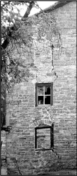
This early 1960s photo of the mill shows one of the many problems, a crack extending almost bottom to top along the south wall of the mill.
